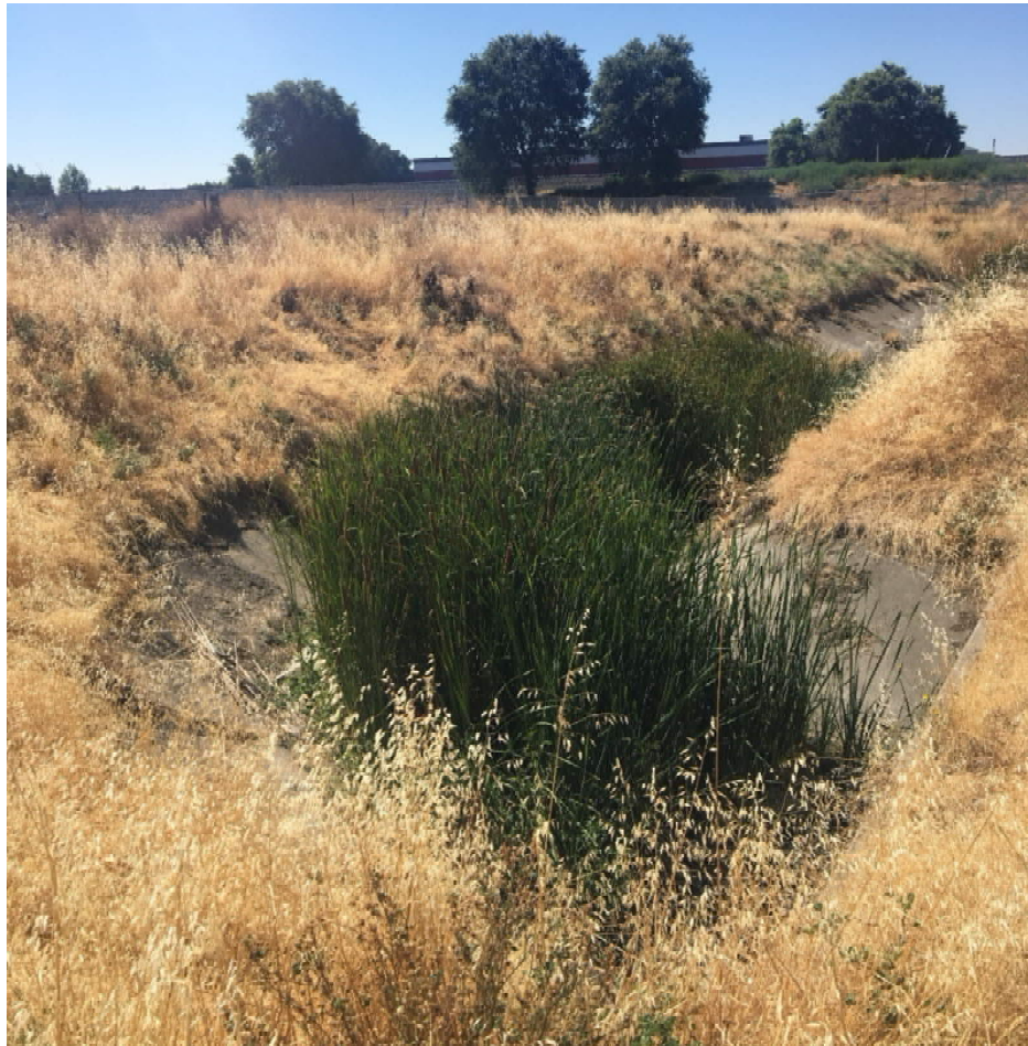
Photo 10-4. RD537/RD811 Channel – Heavy vegetation and mild sedimentation were observed upstream of Jefferson Blvd.
