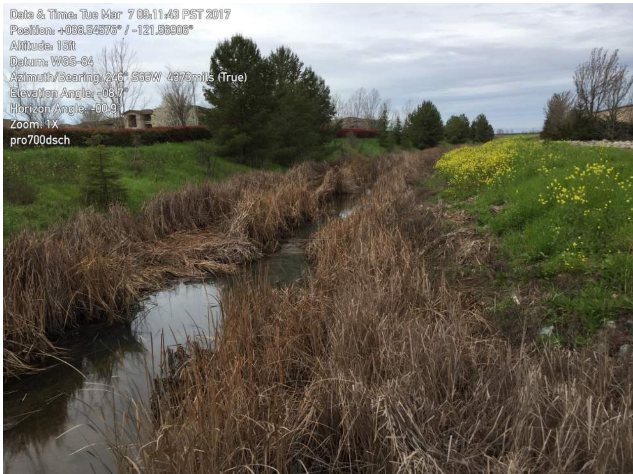
Photo 10-7. SIP Parkway Channel – Typical Vegetation Conditions
