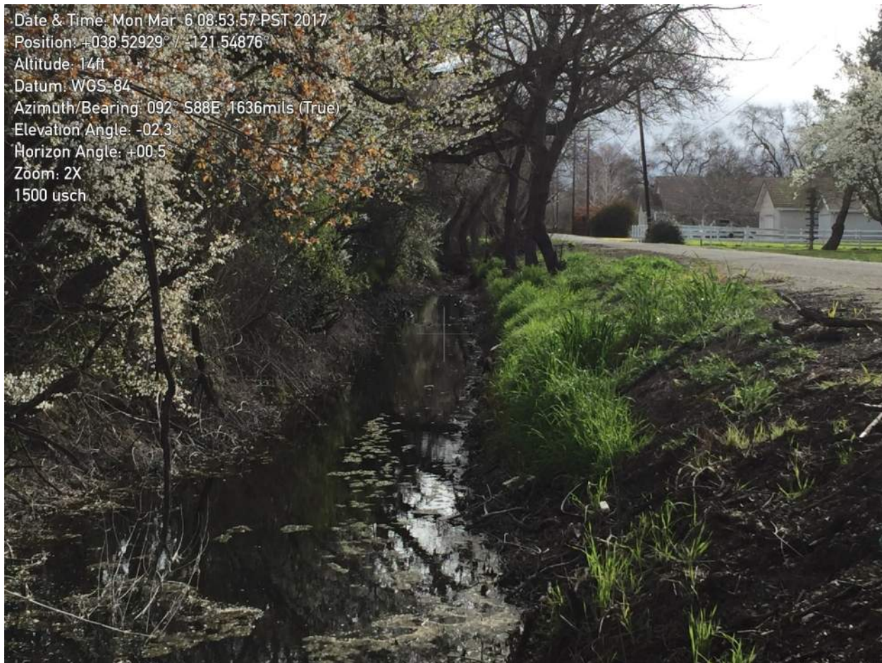
Photo 10-9. Tapley Drain – Typical Conditions Upstream of Partridge Avenue
